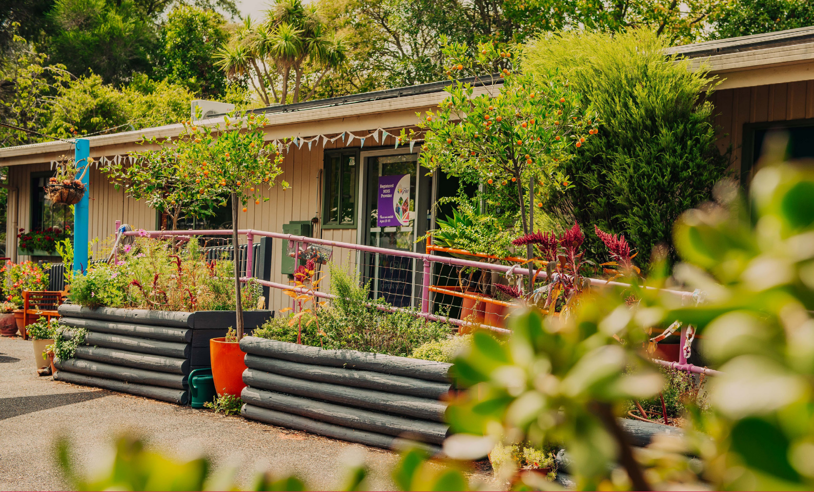
Front entrance at Doncaster
